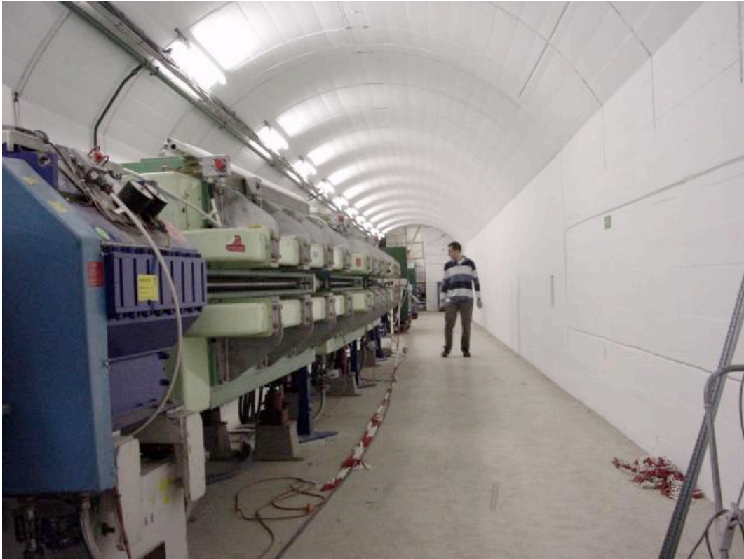
Figure 1.4: Picture of the FTN transfer line installed in the TT2-A tunnel.
