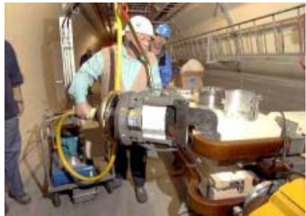
Figure 3 Cutting the dipole magnet excitation bars with a hydraulic nibbler
