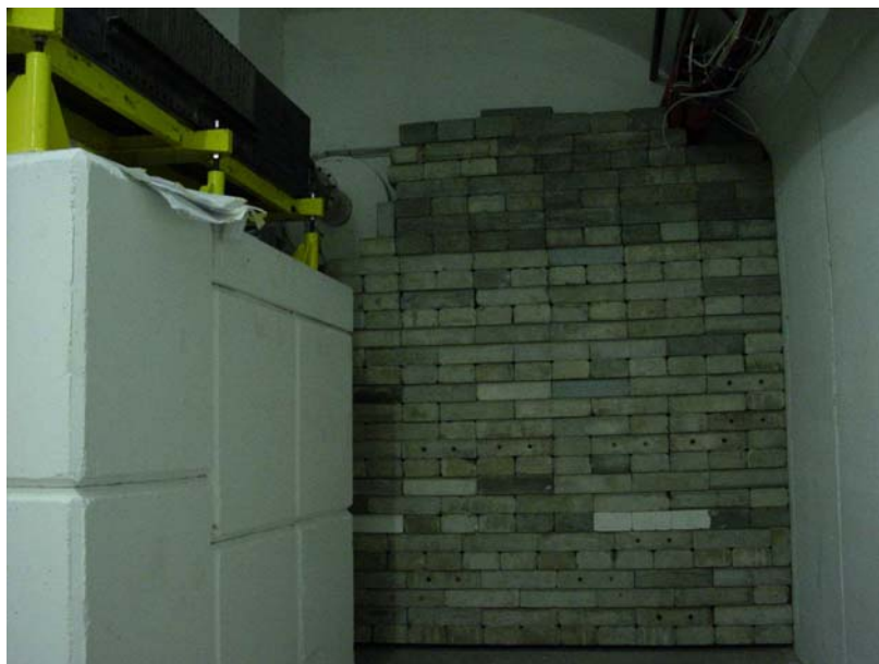
Figure 1. The 40 cm thick concrete wall mounted between the second collimator region and the experimental area.
