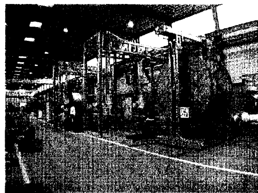
Fig. 2. Construction of the Continuous Electron Beam Welding Plant for the CMS conductor reinforcement.
