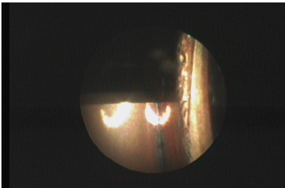
Figure 3: Damaged coupler iris, looking from the beam axis towards the coupling aperture. The section continues to the right.
