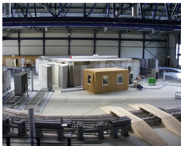
Figure 1: Status of the inside of the building as of March 99, showing the assembled girders, cooling pipes and cable trays. Furthermore the shielding around the microtron and the provisional control room for the commissioning of the injector can be observed.
