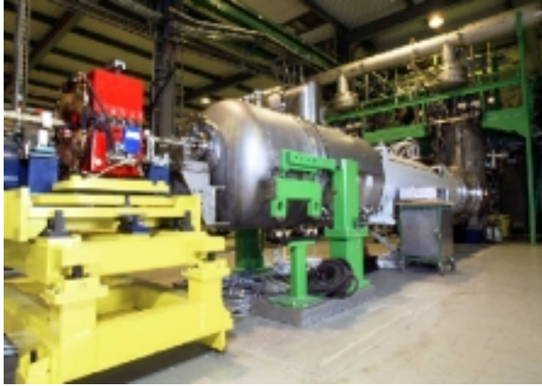
Figure 2: The SSS3 Short Straight Section mounted to cryogenic test station at CERN.
