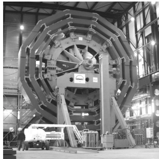
Figure 11: Assembly of the barrel yoke in the CMS surface building.
