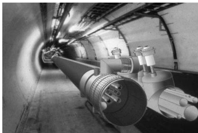
Figure 2: LHC tunnel (CERN photo)
