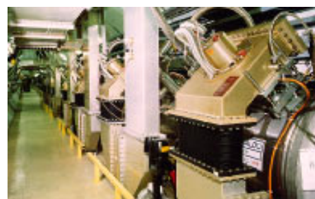
Figure: 2 Couplers mounted on LEP2 modules
