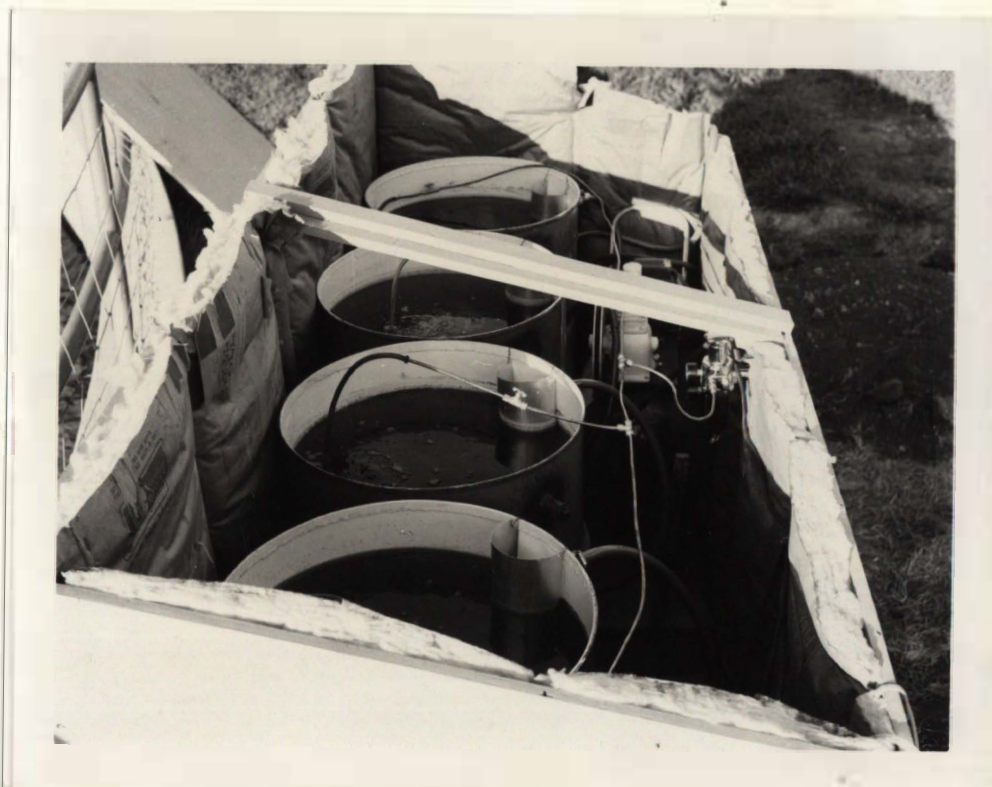
Figure 9. Top view of pilot plant equipment assembled in insulated enclosure.
