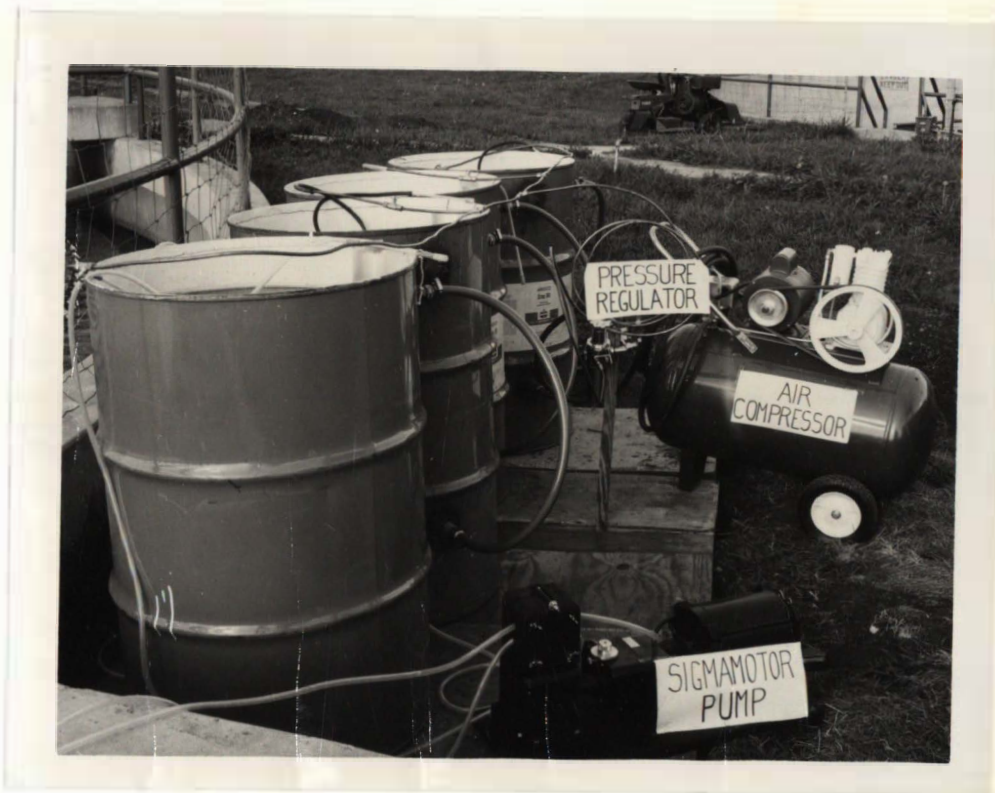
Figure 8. Side view of pilot plant equipment.
