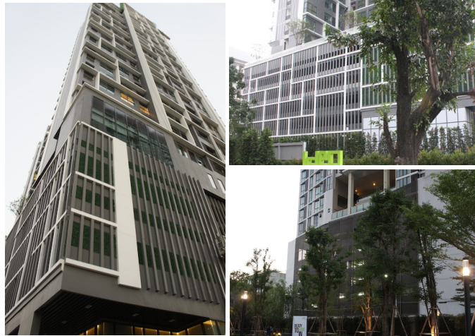
Figure 2 Exterior of the Ideo Mobi Sathorn condominium
