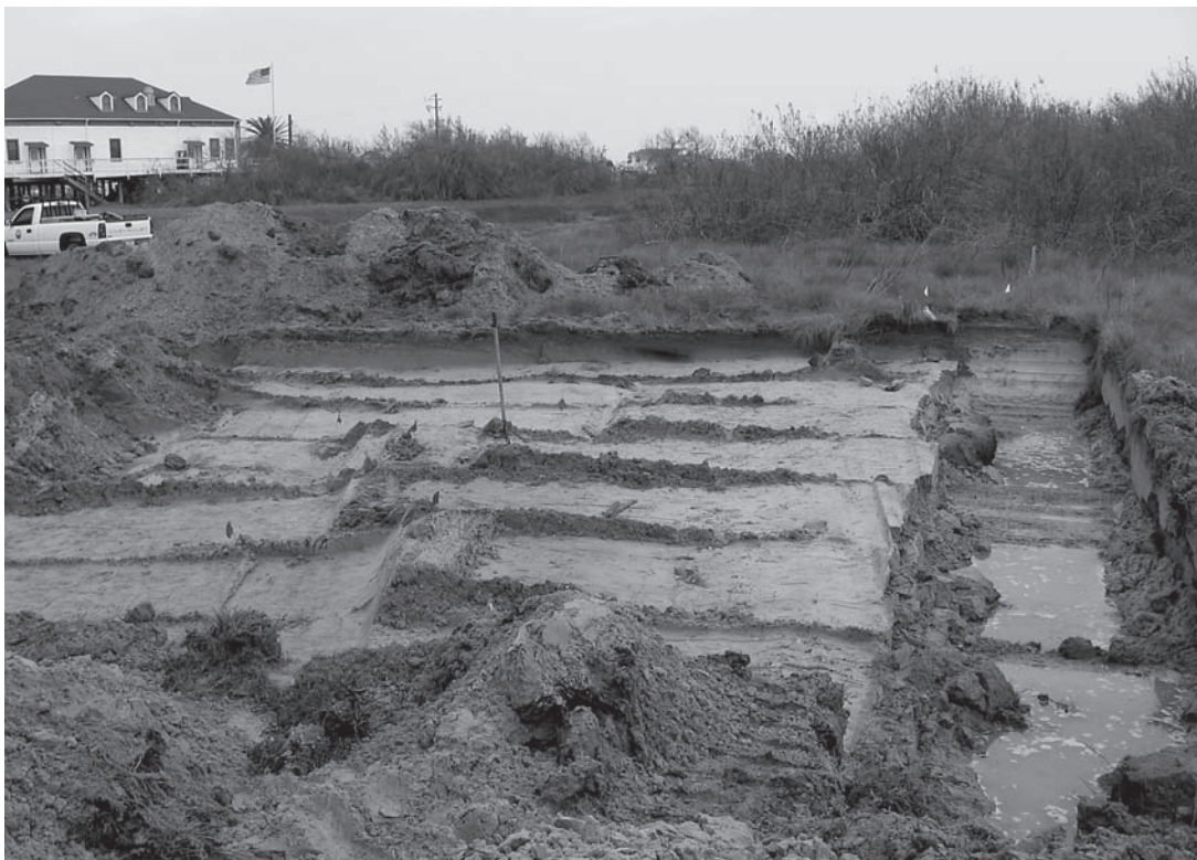
Figure 3.5. View of the block excavation formed by contiguous gradall trenches, looking eastward down Trench 17 (partially filled with water on right). Surfside Beach City Hall is in the background on the left.
