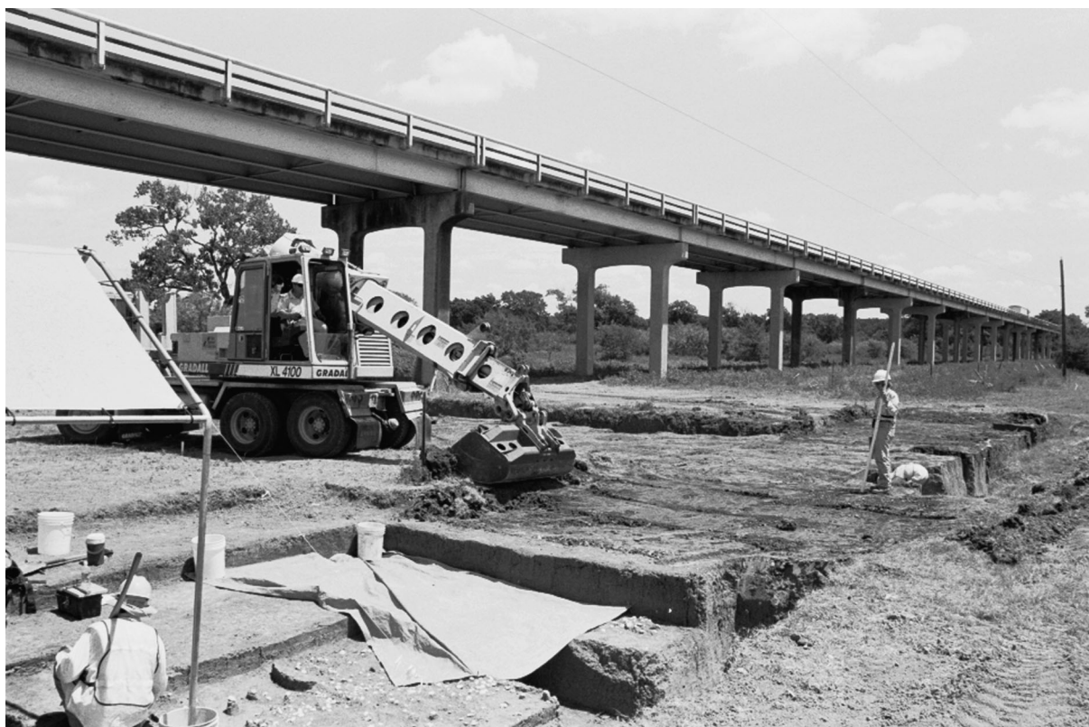
Figure 4-3. View of a TxDOT Gradall stripping the area where the East and South Blocks eventually would be opened as excavations in the Main Block begin.
