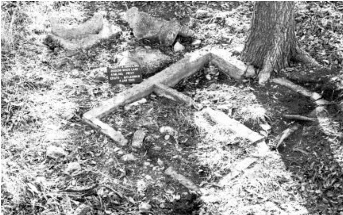
Figure 15. Photograph of concrete privy foundation at the Erath/McLennan House, 41ML140. View is southwest.
