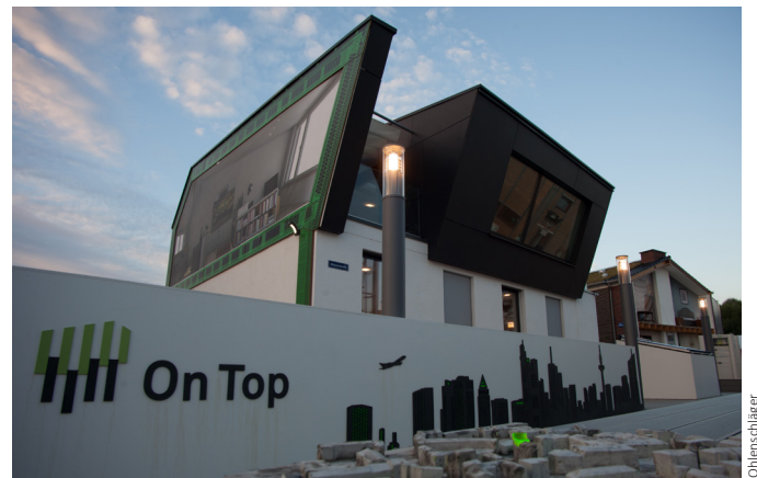
Construction “OnTop” at Solar Decathlon in Versailles.
