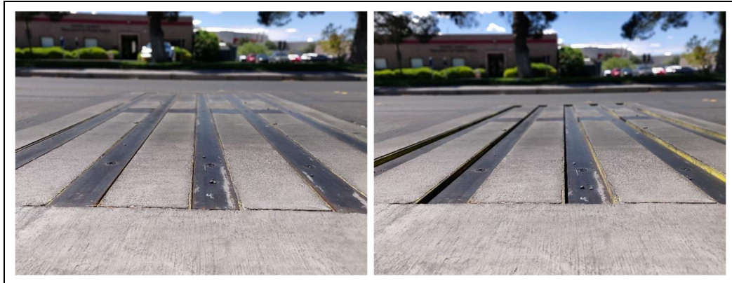
Figure 5. Inactive (left) and active (right) states of DRTRS.
