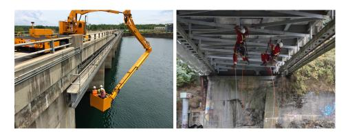
Figure 4.1: Structures inspectors working at high altitude.
