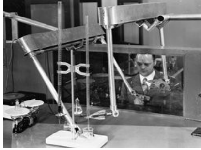
Figure 5 Goertz's mechanical slave-master manipulator [25]
