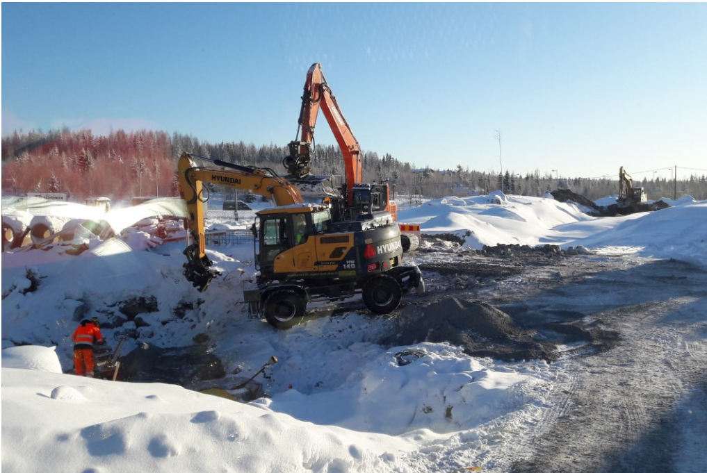
Figure 10. Work in progress at a construction site.
