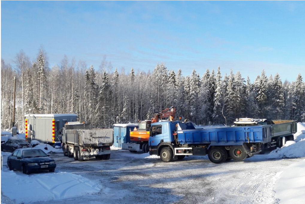
Figure 9. Trucks parked at a construction site office during lunchtime.
