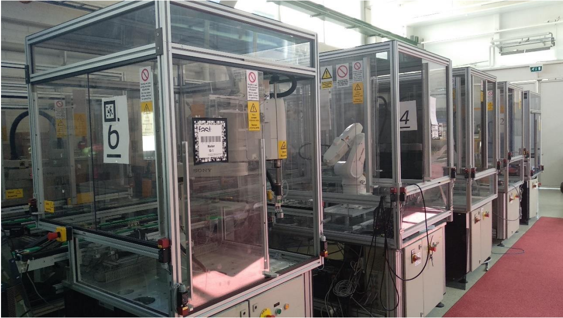
Figure 29. FASTory production line
