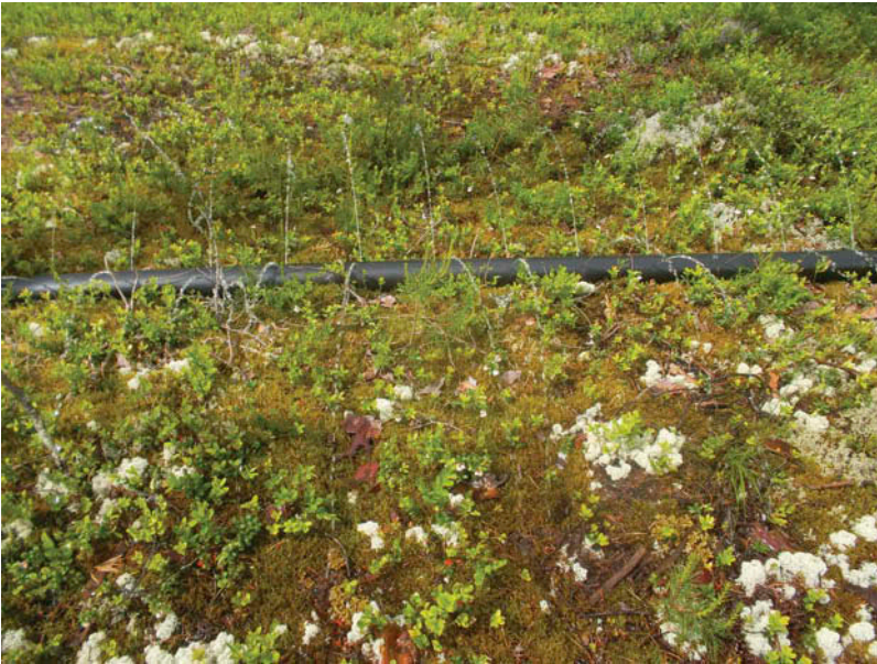
Figure 5. The sprinkler system consists of perforated pipes.
