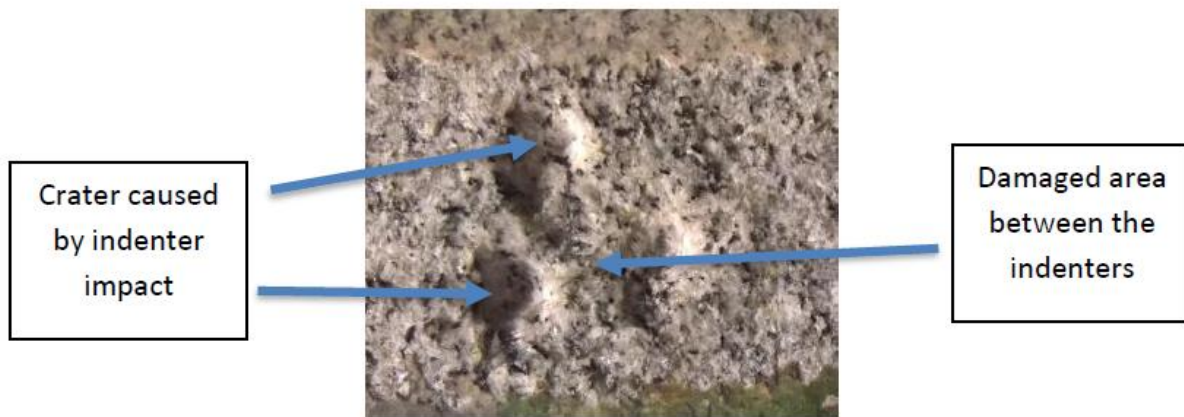
Figure 7 Damaged area on a 6-second heat shocked sample
