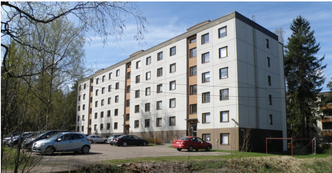
Figure 7. A typical precast 1970s slab block.
