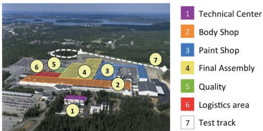
Figure 45. Aerial view of the case company with production department locations.
