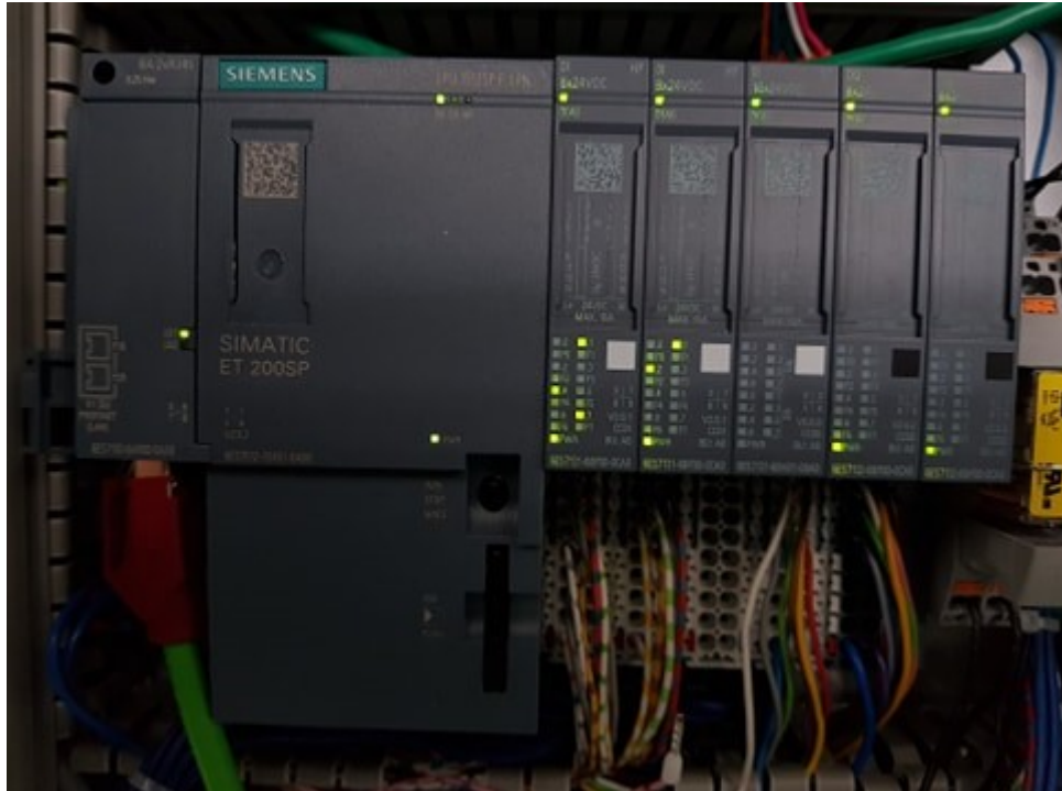
Figure 20 ET200SP Module- Distribution Station
