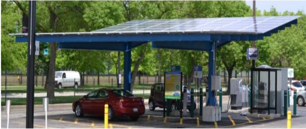
Figure 4.10 Solar panels and charging stations at IIT [36].
