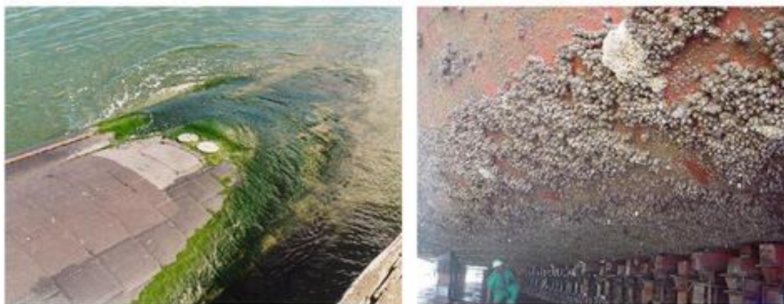
Figure 13. Classical examples of biofouling in structures having somewhat continuous water contact. Adapted from (Callow & Callow, 2011)
