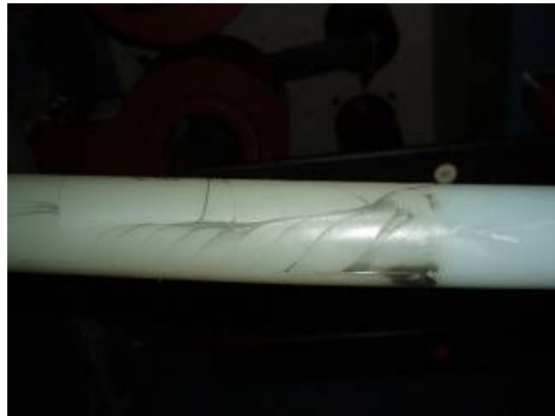
Figure 3.1. Surface tracking on top of insulation [25]
