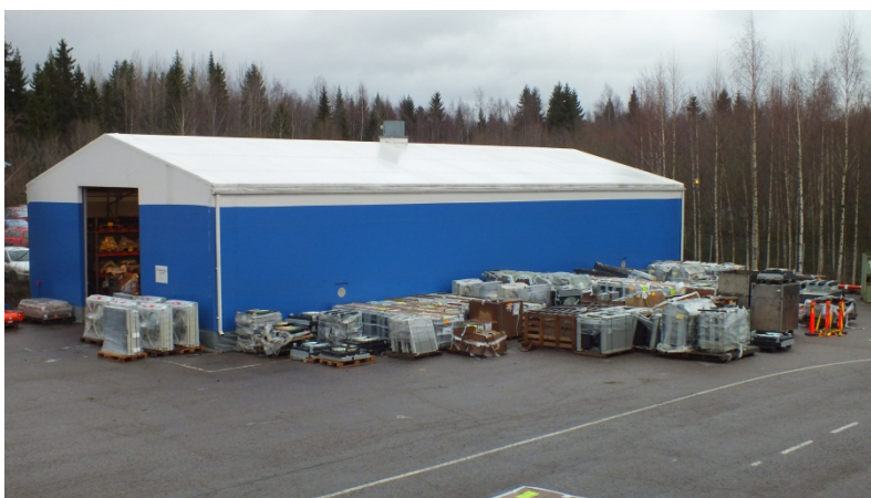
Figure 8: SF storage tent pictured from MP3-building.
