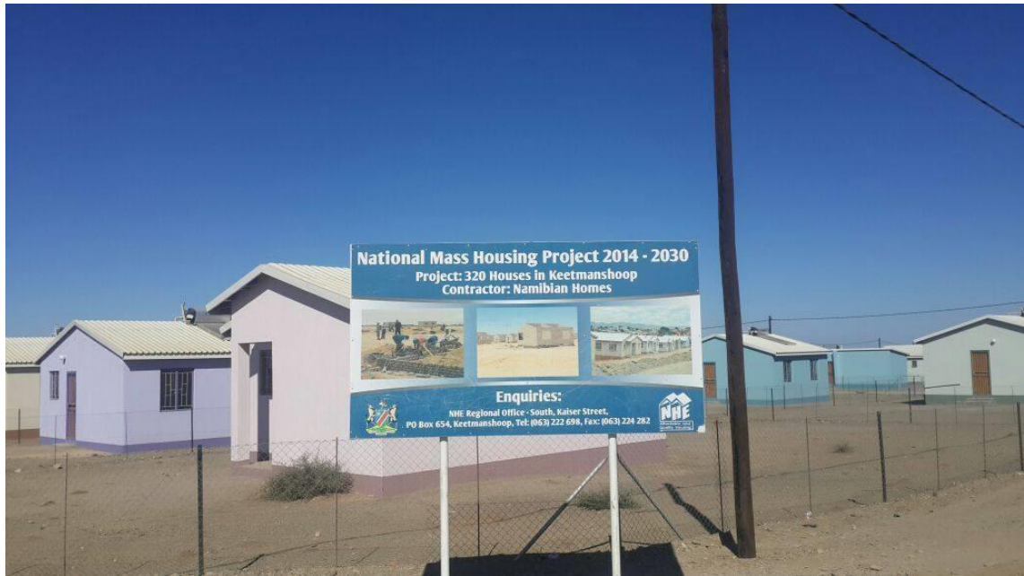
Fig. 5-11. National Mass Housing Project in Keetmanshoop (Salmivirta 2015).
