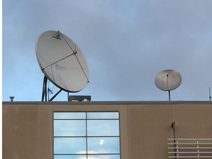
Figure 11. Parabolic antennas in TUT.
