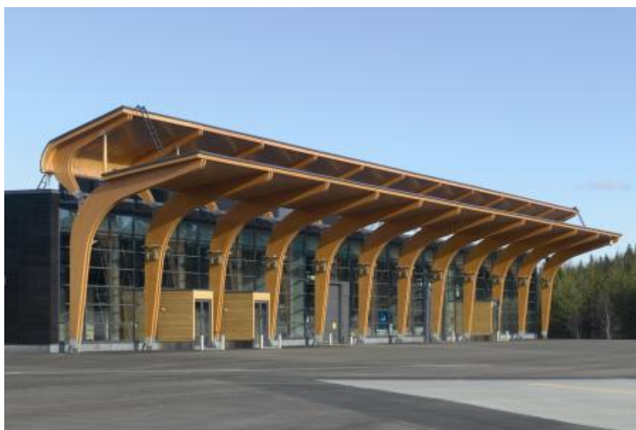
Figure 3.42 Glulam (GL) structures in the airport terminal in the city of Jyväskylä (Source: Late-Rakenteet Oy)
