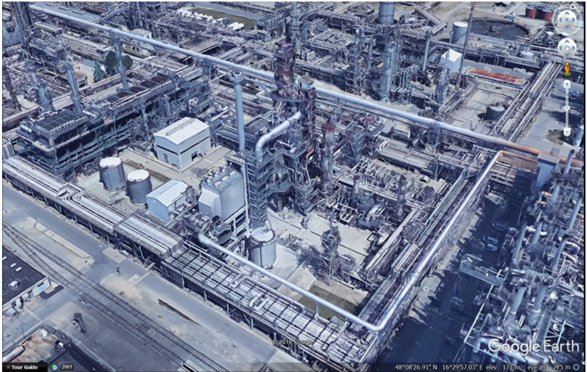
Figure 8. OMV refinery in Schwechat, Austria [45].
