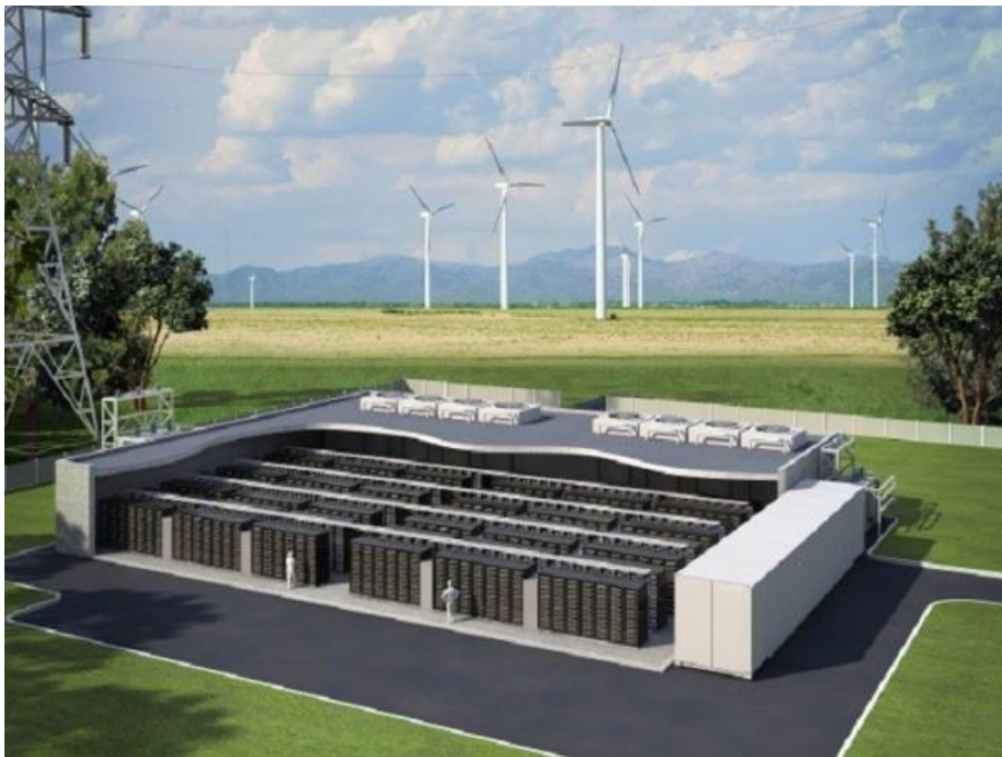
Figure 2-4 Energy storages (batteries) installed with wind turbines in Sweden
