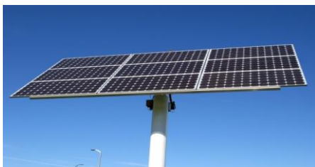
Figure 2-1 Typical solar panel tilted towards sun
