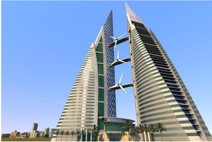
Figure 3-2 Horizontal axis wind turbines installed between two buildings of world trade center located in Bahrain
