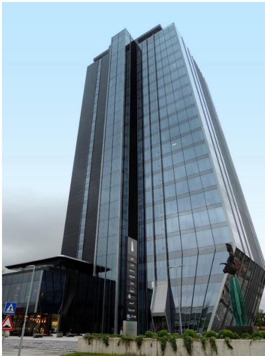
Figure 3-1 PV panels installed in Crystal palace located in Slovenia
