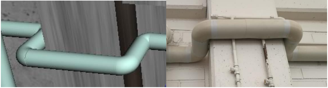
Figure 38. Intersection of two parallel pipes, bypassing a column
