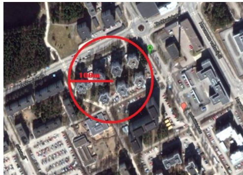
Figure 5.14 Apartment Complex for smart metering.
