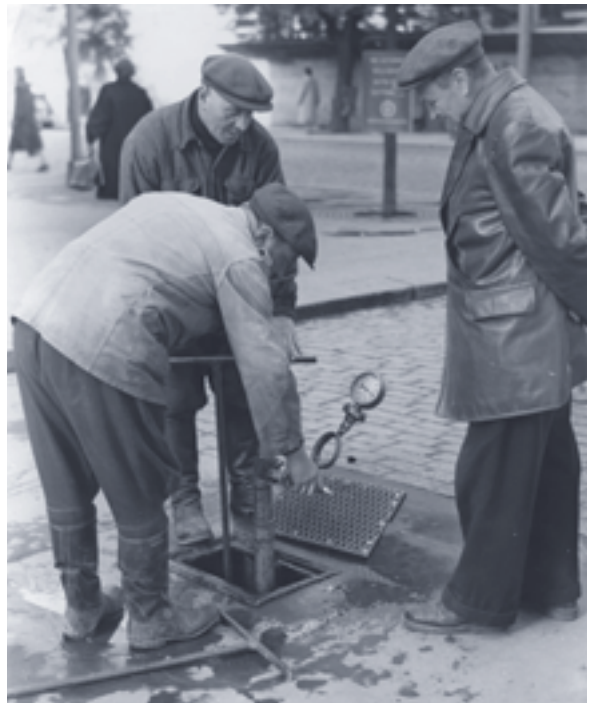
Fig. 4.4 Measuring water head through fire hydrant in the city centre in the late 1940s (Photo: Photo Archives of Tampere Museums).
