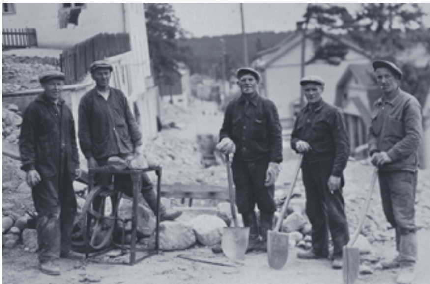
Fig. 9.1 Construction of water pipeline by Pispala water cooperative (Photo: P. Wilén).
