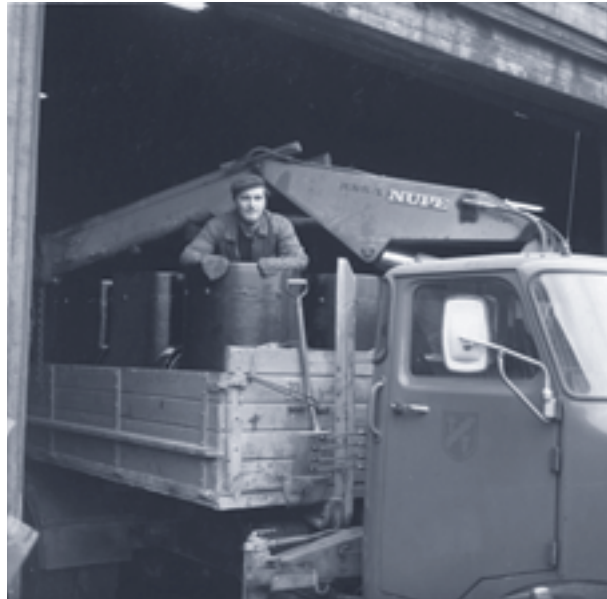
Fig. 7.2 Mr. Pauli Sirén fetching T-pipes of SG cast iron around 1970.
