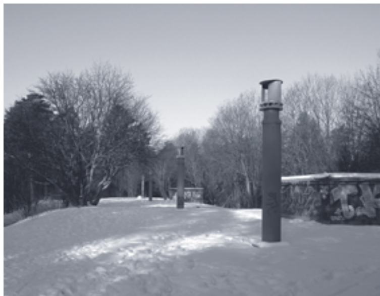
Fig. 4.6 Cross-section of the underground water reservoir in the Pyynikinharju esker taken into use in 1898 (upper: Brandt 1899), and the same facility over 100 years later (Photo: T. Katko).
