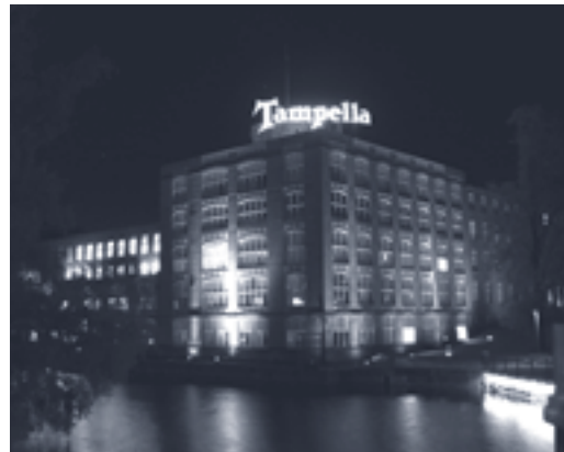
Fig. 6.1 The best known traditional industries in Tampere also in relation to water history: The six-storey industrial building of Finlayson with its originally combined water reservoir and dry toilets (upper), and the Tampella factories with a water reservoir hidden behind the sign (Photos: T. Katko).
