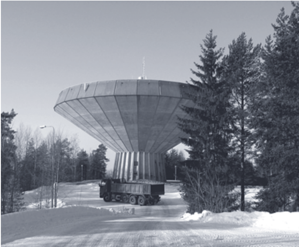
Fig. 4.7 The first mushroom-shaped water tower of Tesoma in the western part of the city, completed in 1969 (Photo: T. Katko).
