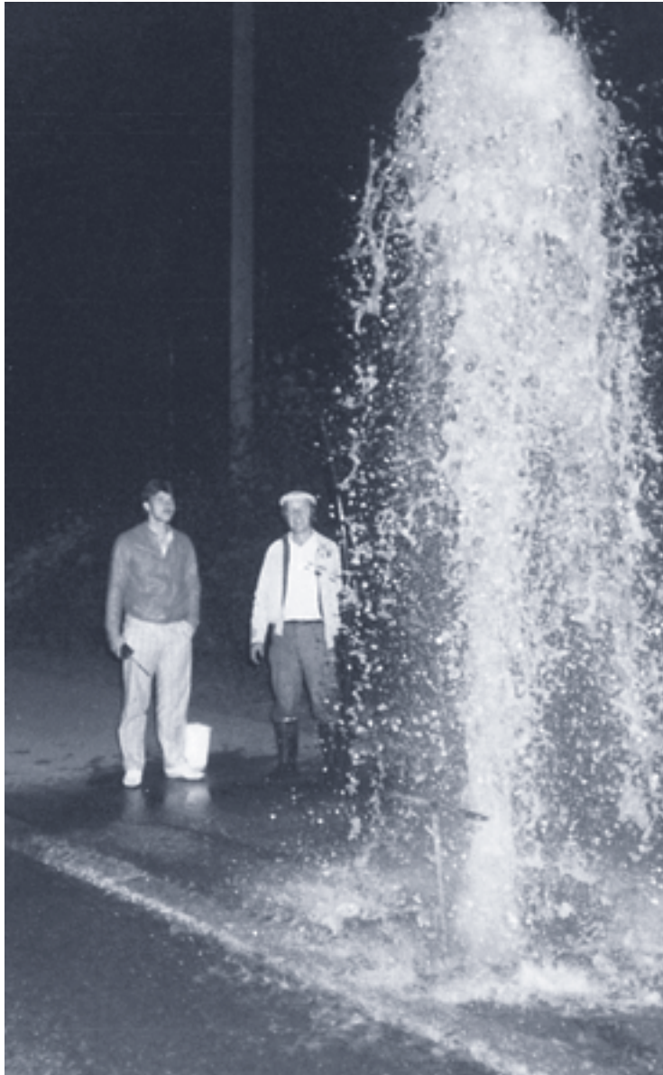
Fig. 4.11 Flushing of water network during a summer night 1986 (Photo: Tampere Water).
