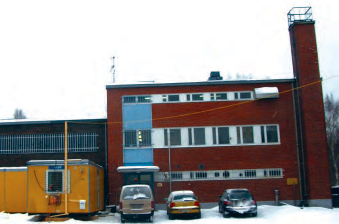
Picture 2a and b. The third ground water intake, with a ground reservoir holding 700 cubic metres, was completed in Herajoki in 1963. (Juuti 2009)
