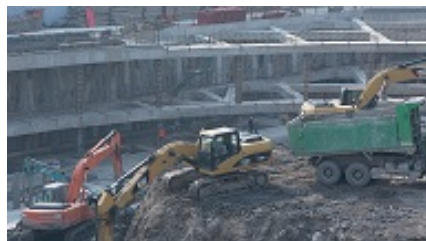
(b) Construction Field.
