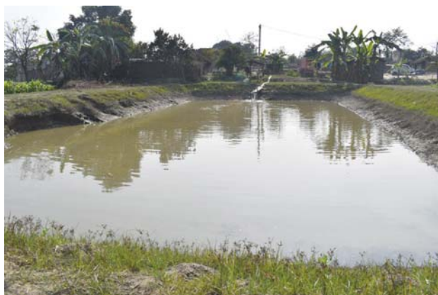
Fig. 11.4. Water harvesting structure for irrigation and fish farming
