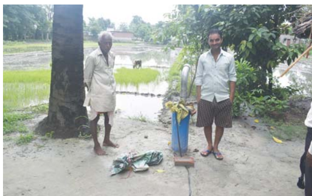
Fig. 11.5. Borewell installed at farmer's field for irrigation
