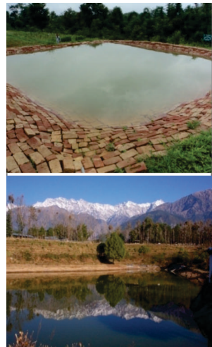
Plate : Poly-lined tanks for rain-water harvesting in hills
