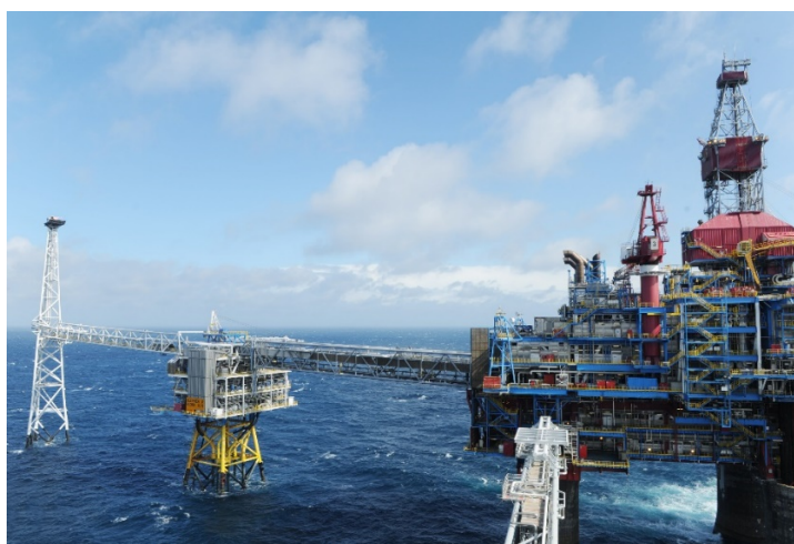
Figure 9. The Sleipner platform with the CO 2 separation unit in the centre (Source: Statoil)
