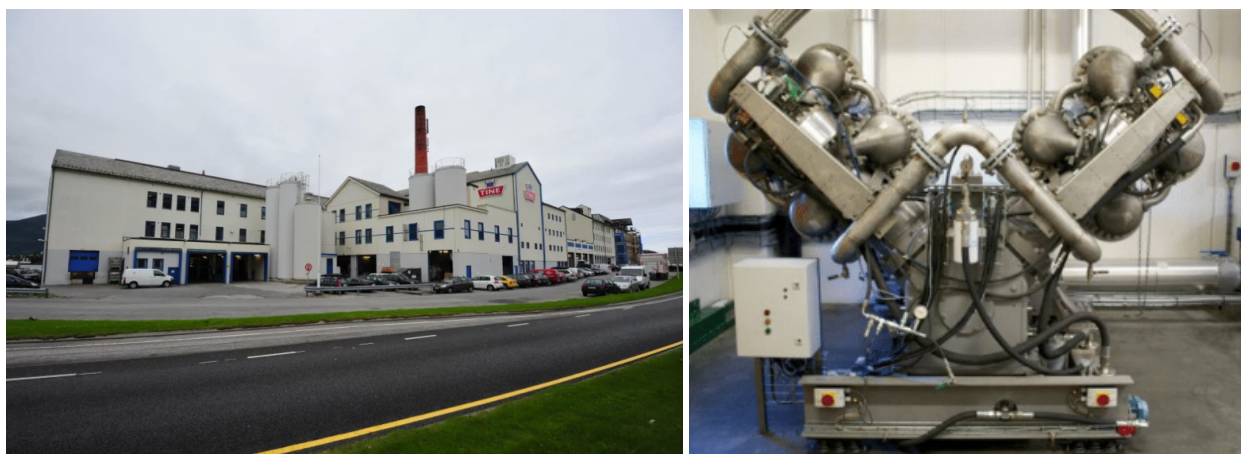
Figure 5: (Left) Tine facilities in Ålesund (NO); (Right) HTHP unit from Single Phase Power – Photos: Tine SA.
