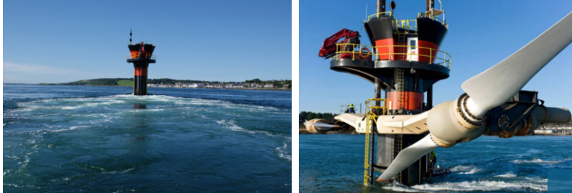
Figure 4.1: Wake behind the SeaGen monopile in Strangford Narrows (Northern Ireland, UK) (left) and blades that are out of water (right)
