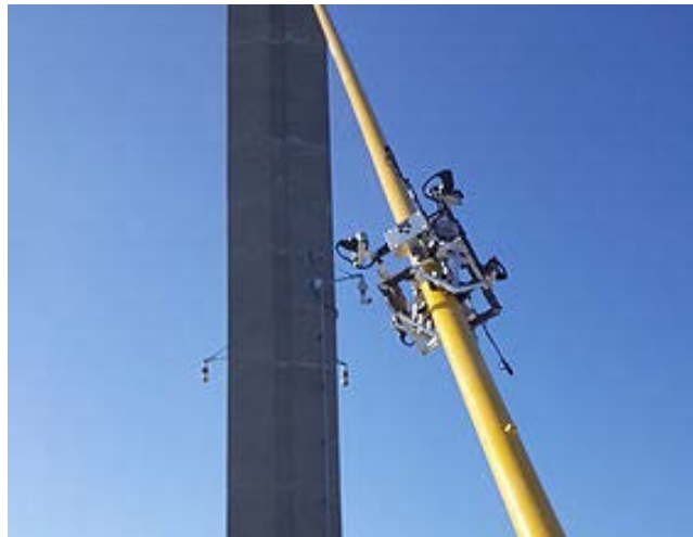
Figure 1: IPC CableScan - Robotic Cable Stay Inspection. Credit: IPC
