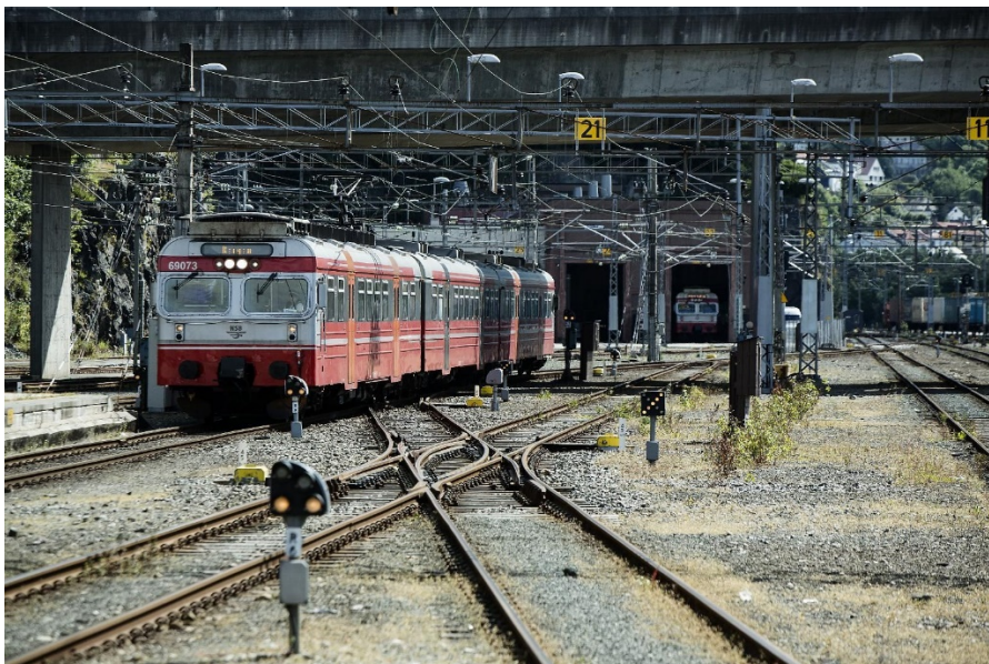
Figure 3: Railroad Infrastructure between Bergen and Fløyen. Credit: Silje Katrine Robinson
