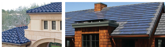
Figure 1: Examples of BIPV tiles on building roofs, Solar Thermal Magazine [1] and Applied Solar (right) [2].
