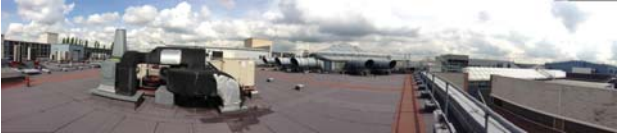
Figure 21 – Brent Cross Shopping Centre Roof
