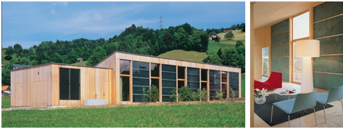
Fig. 1. On the left; External view of building with a combination of standard windows and PCM-windows (Architekten, 2000a). On the right; internal view of standard windows and PCM-windows in combination, PCM being the semi-translucent elements on the sides of the windows (Architekten, 2000b, 2004).
