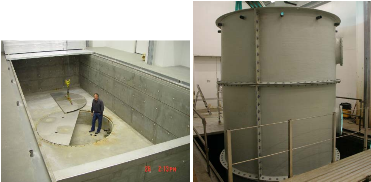
Figure A.1: Ice basin without propellers and other equipment used for circulation showing the fundament for the Tower Basin (left) and the initial mounting of the Tower Basin in January 2011 (right).
